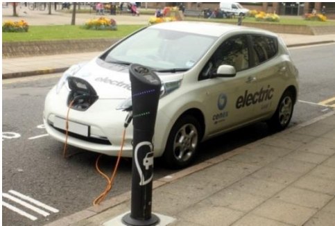
Figure 12 - Conductive charging post
