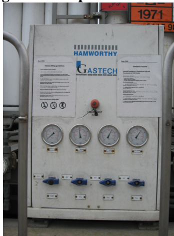
Figure 5 - Dispenser valve unit
