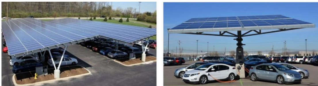
Figure 19 Solar PV Canopy Configurations 20
