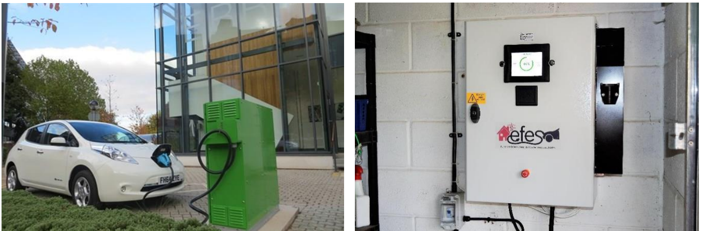
Figure 17 Prototype V2G Units - Commercial Building (left) and Domestic Building (right)
