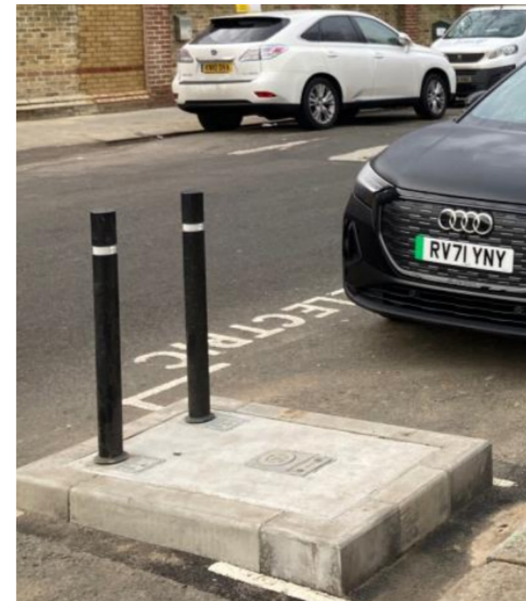
A NAL socket awaiting a chargepoint in an on-street location
